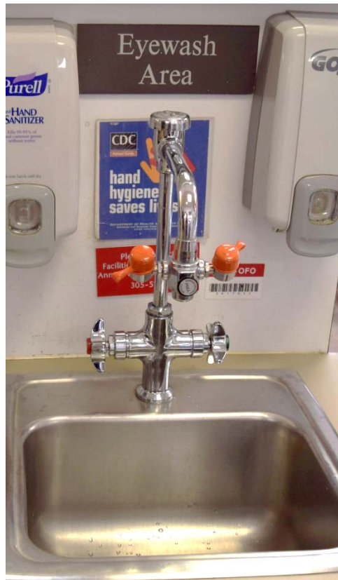
Eye Wash Station
