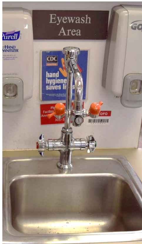
Eye Wash Station
