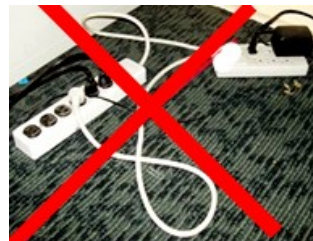
Photo shows prohibited "Daisy Chaining" - one power strip connected into another.
