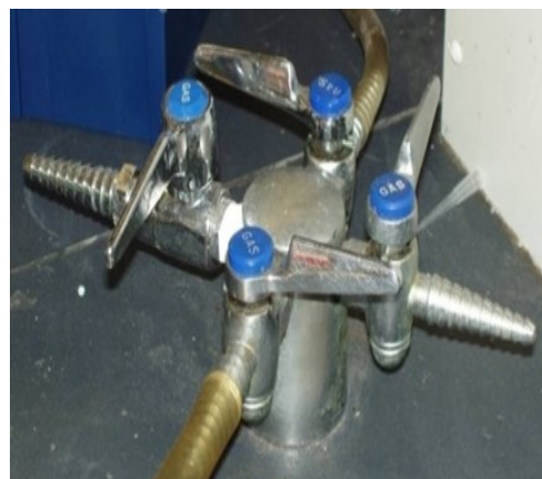
Turn valve clockwise to close To close, make sure lever is perpendicular to
