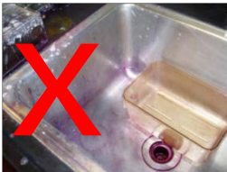
Stained sink due to drain disposal
